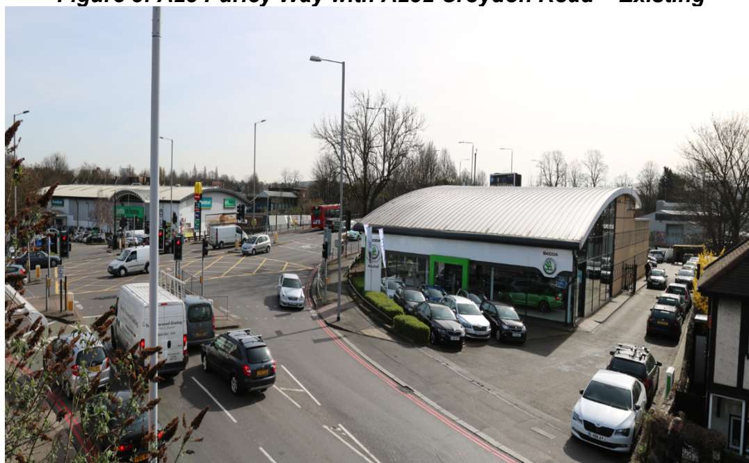
Figure 3: A23 Purley Way with A232 Croydon Road – Existing
